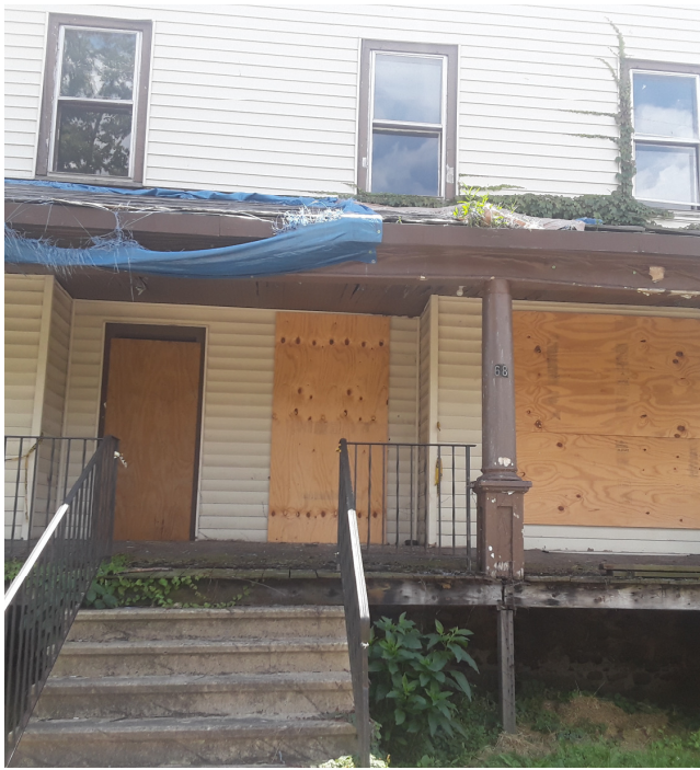
Front of Building (Side A)
