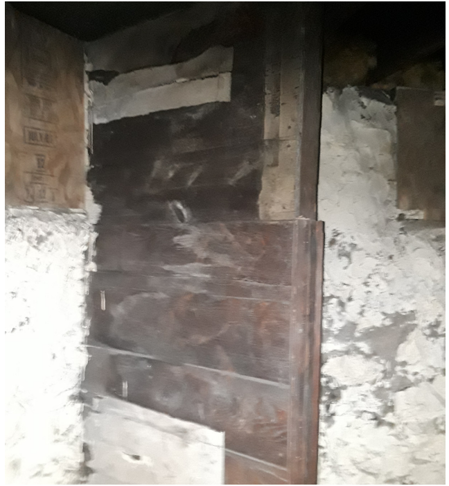
Basement 14 - Positive wood wall
